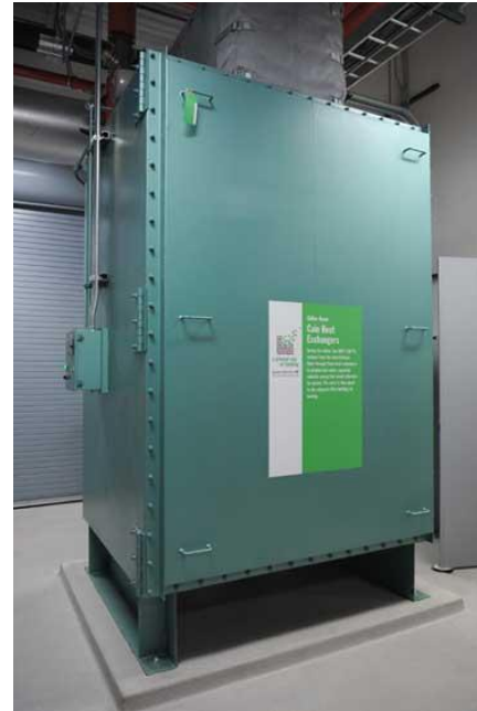
Exhaust to Hot Water HEX
