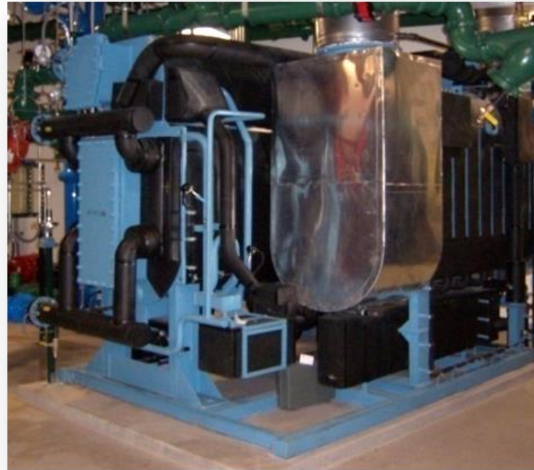
Exhaust Fired Double Effect Absorption Chiller
