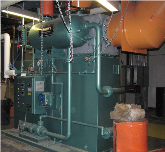
Heat Recovery Steam Generator
