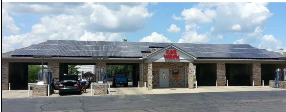
SJ Kuss Car Wash, Canal Winchester, OH 18.4 KW solar system on shingled roof
