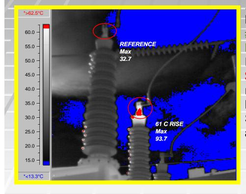
ROI CASE STUDY... Large US Utility #3A Bank 220/66 KV Hot Bushing Rod Potential loss – \$2,000,000 (based on previous failure and repair). Because fault was found, they were able to Schedule repair @ \$15,000 (includes parts
