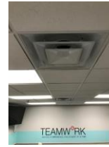
Supply air diffuser
